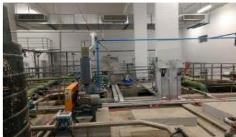
Sewage Treatment Plant
