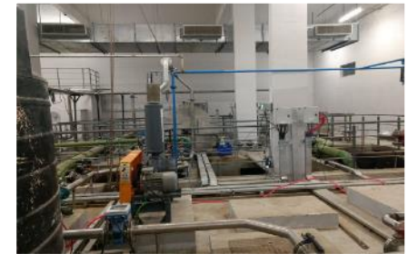
Sewage Treatment Plant
