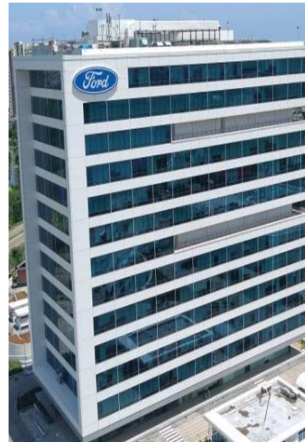
High Performance Glazing System - Façade
